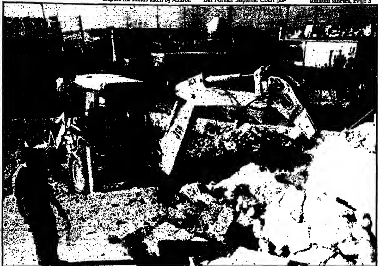
A municipality demolition crew finishes razing an illegally built center for the disabled in eastern Jerusalem yesterday.
